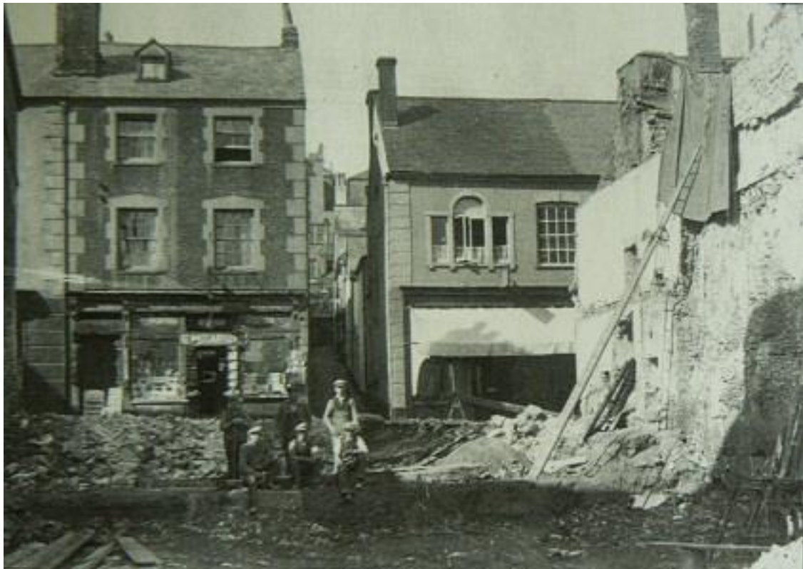
Demolition of the Steam Packet Hotel in 1937.
